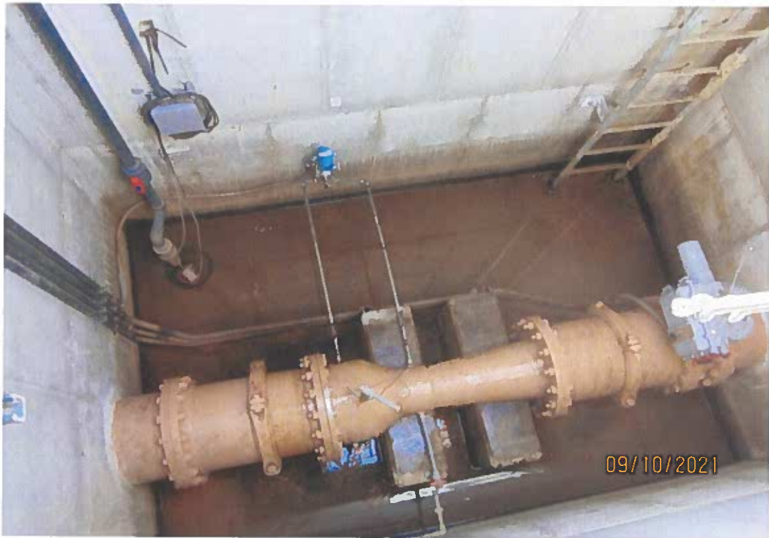
Photograph I - Influent Flow Meter Vault
