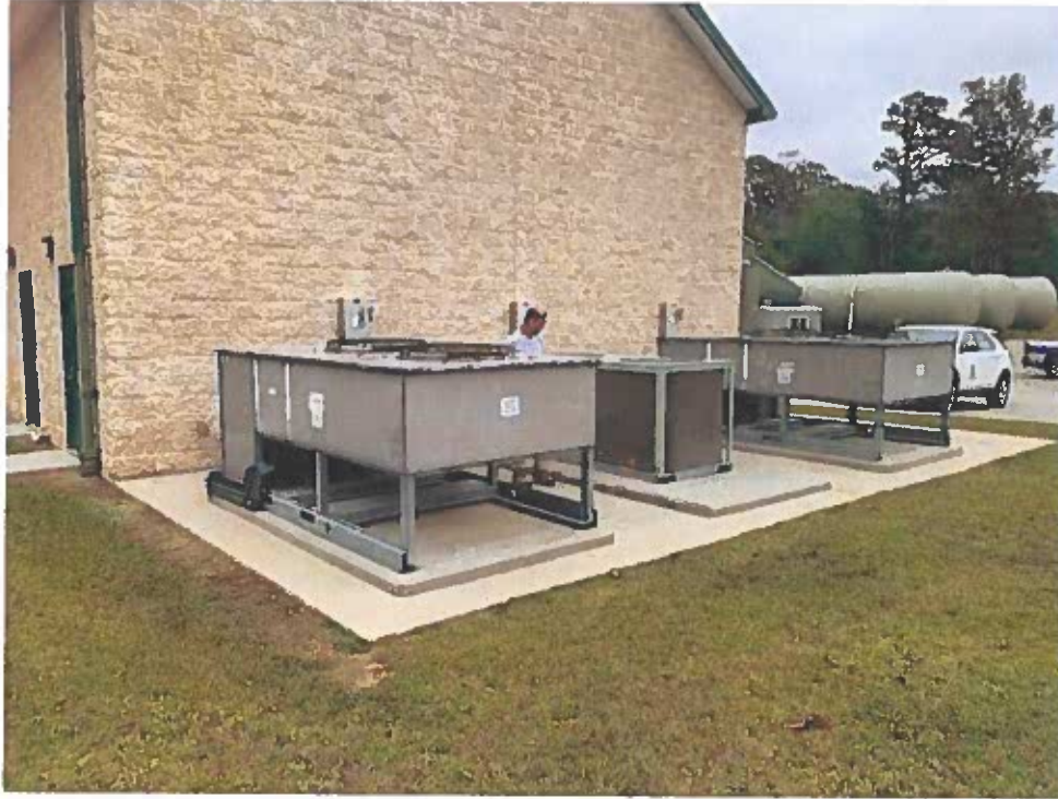
Photograph E – New HVAC unit for Electrical Room
