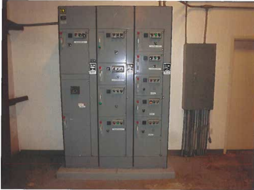
Photograph Q – Breaker Panel in Generator Building
