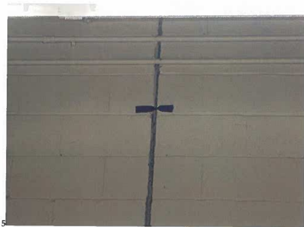
Photograph C – Existing Crack in Electrical Building Wall
