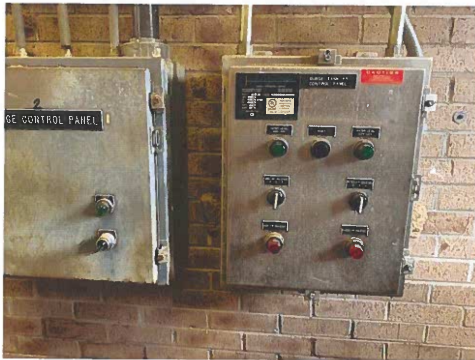
Photograph L- Surge Tank 3 Control Panel Power Off
