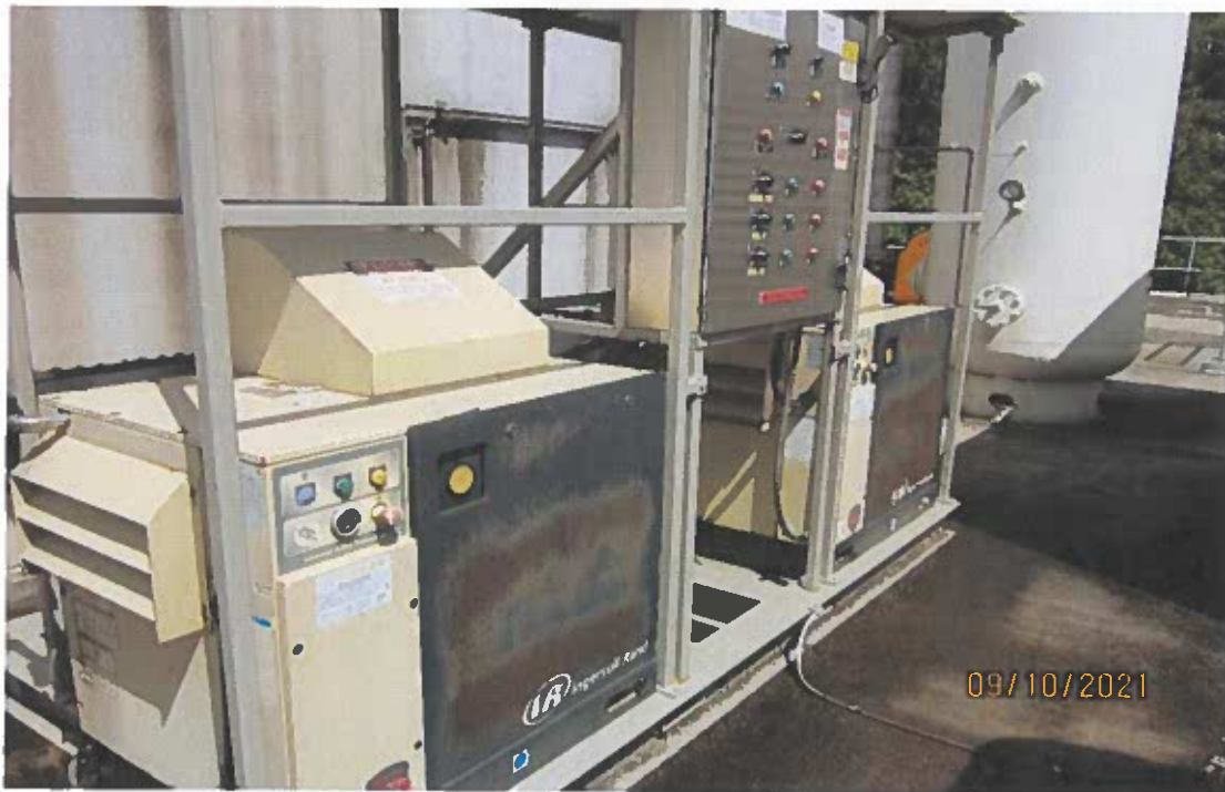
Photograph H – Restored air compressor skid support framing
