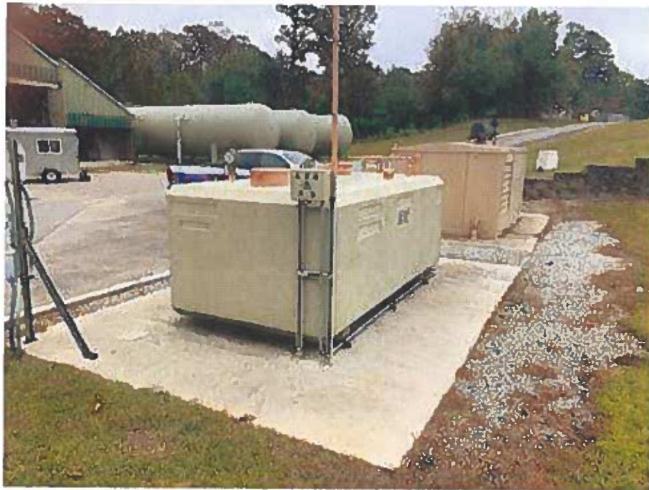
Photograph J - Small Generator and Tank
