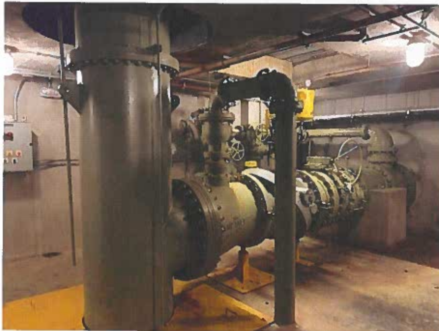
Photograph B – Spare Check Valve on Pump
