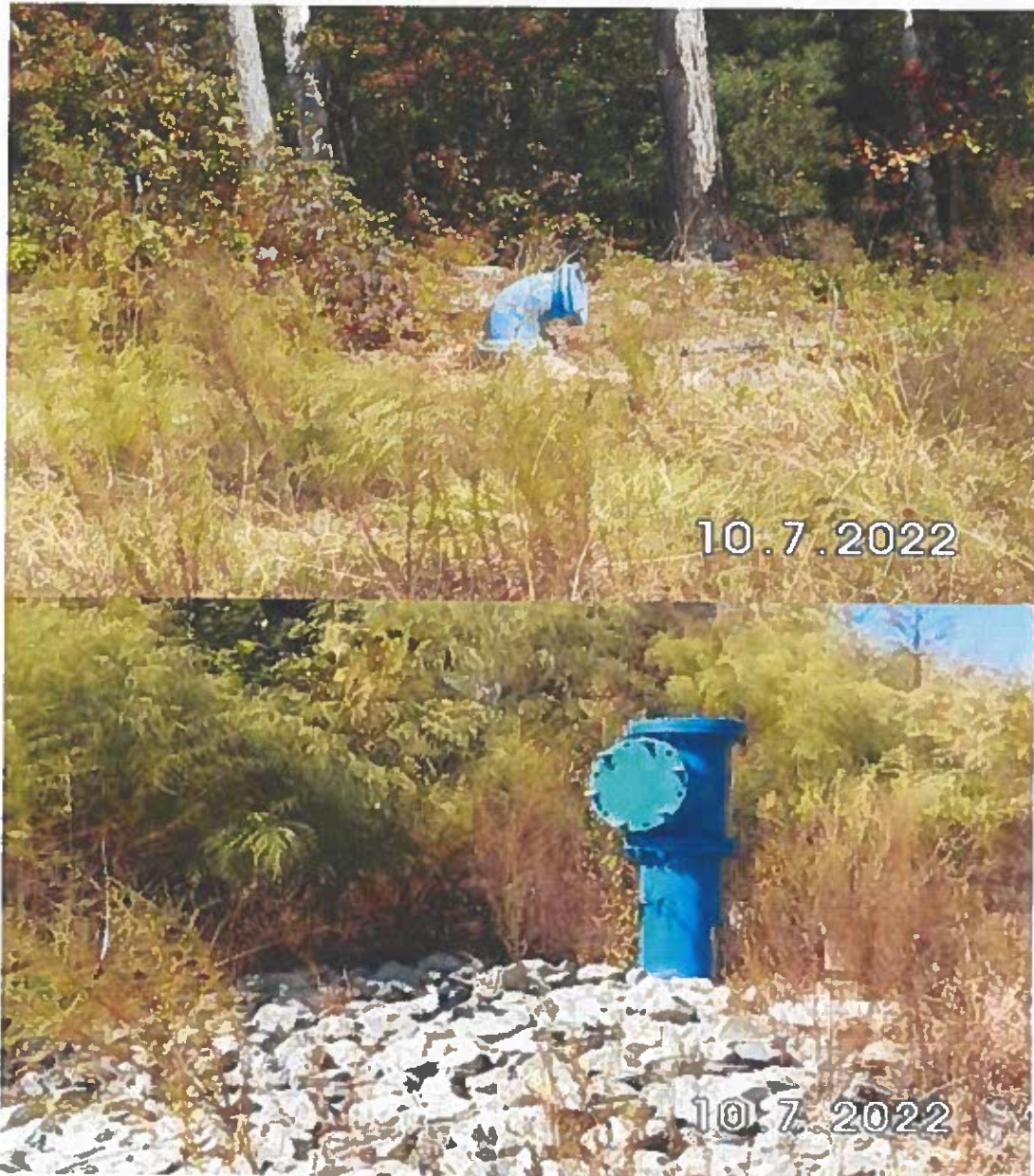
Photograph GG- Old Blow-off on 48" RWM and new Blow-off on 54" RWM
