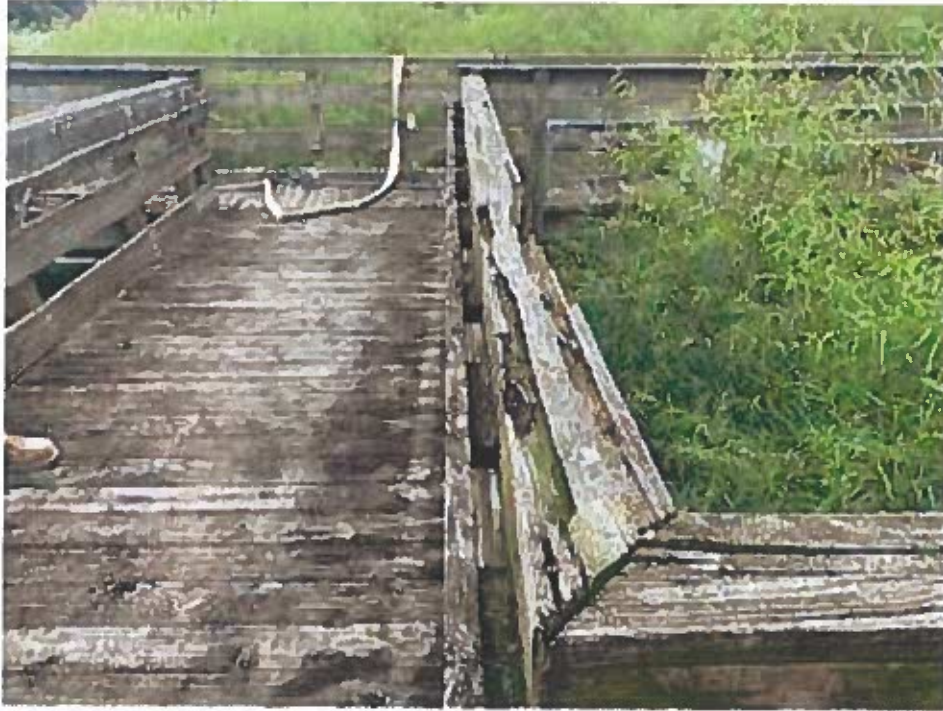
Photograph O – Failed Handrails near New Backwash House
