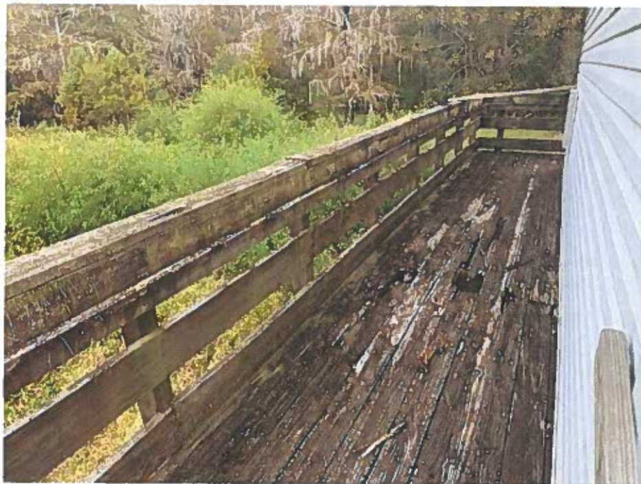
Photograph N- Failed Deck Adjacent to New Backwash House
