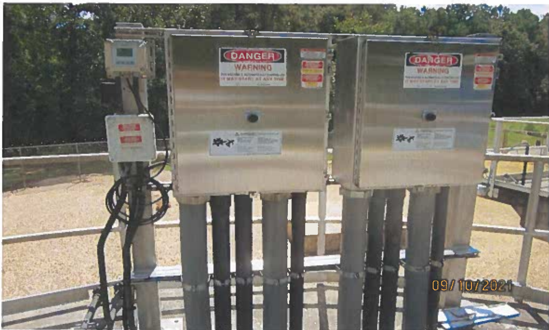
Photograph E – Intake Pump Station Controls Station
