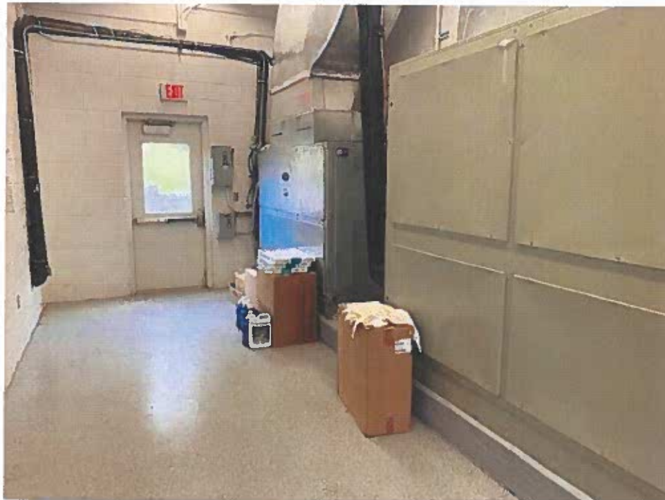
Photograph F – New HVAC Air Handling unit
