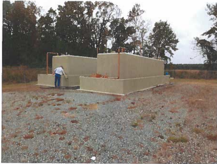
Photograph G – Diesel Fuel Storage Tanks
