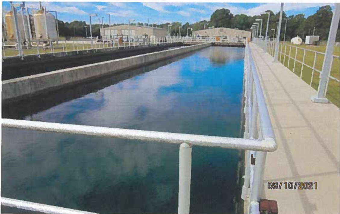
Photograph J - Sedimentation Basins
