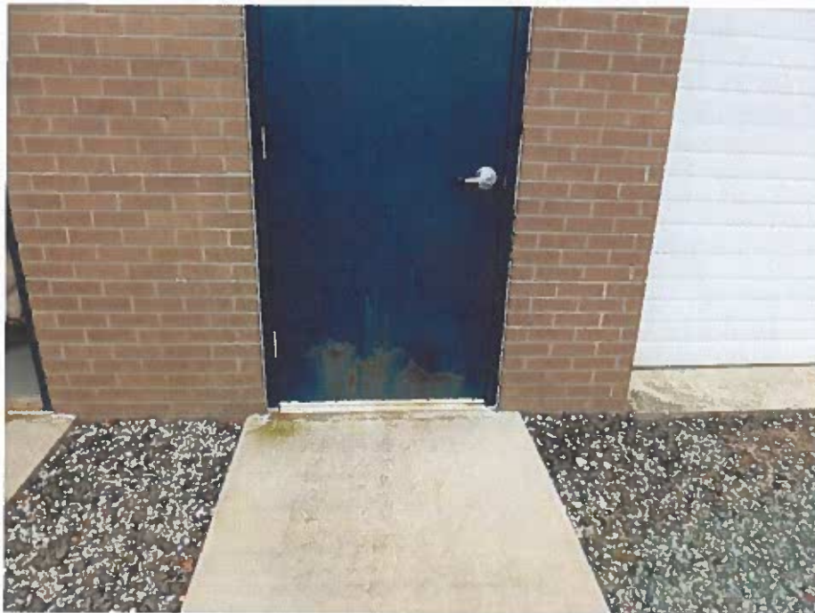
Photograph P – Corroded Personnel Doors at Generator Bldg
