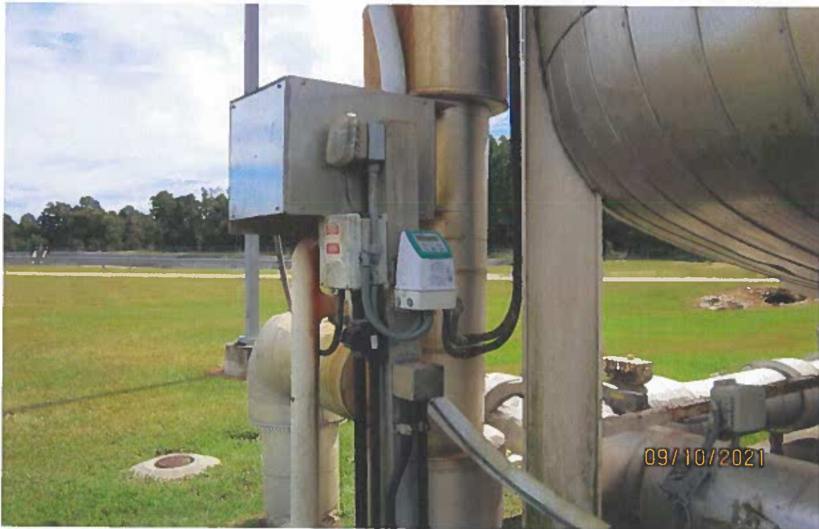
Photograph O – Flow Meters at GAC Filters
