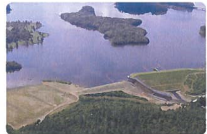
Hard Labor Creek Regional Reservoir Dam
