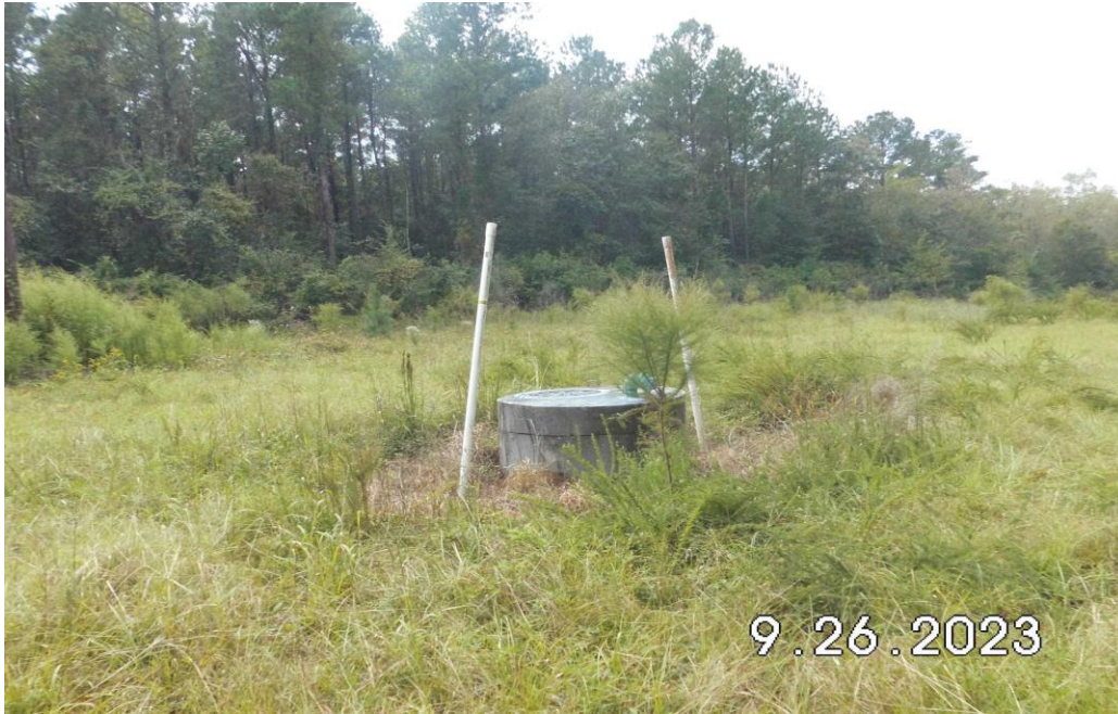
Photograph BB – Orange Painted Structure Marker Deterioration
