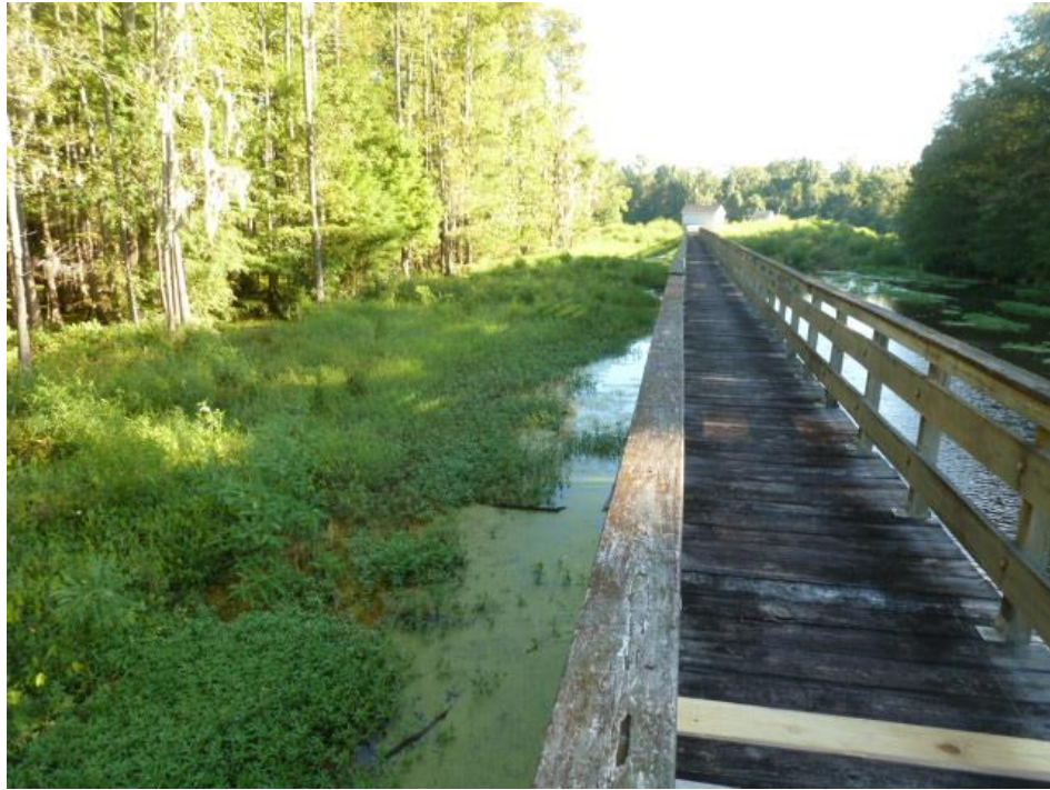
Photograph O – 60-inch Intake Pipeline Corridor
