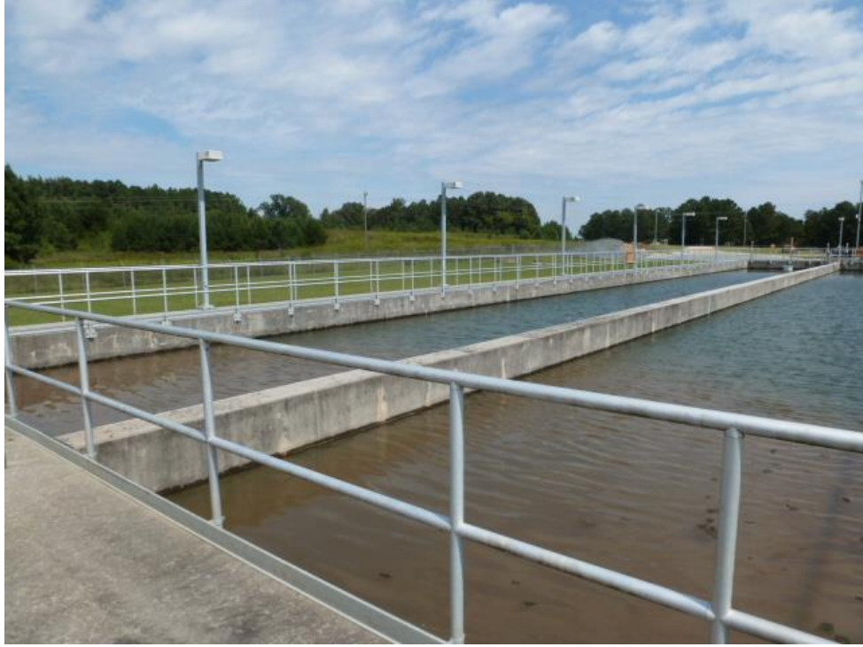
Photograph M – Sedimentation Basins
