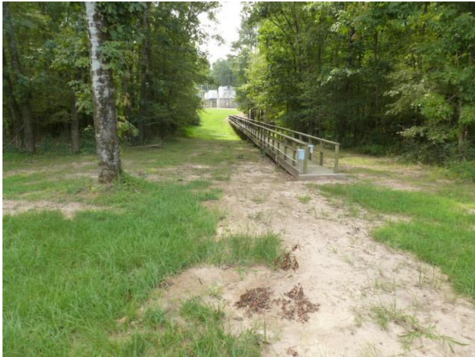
Photograph D – River Access Walkway
