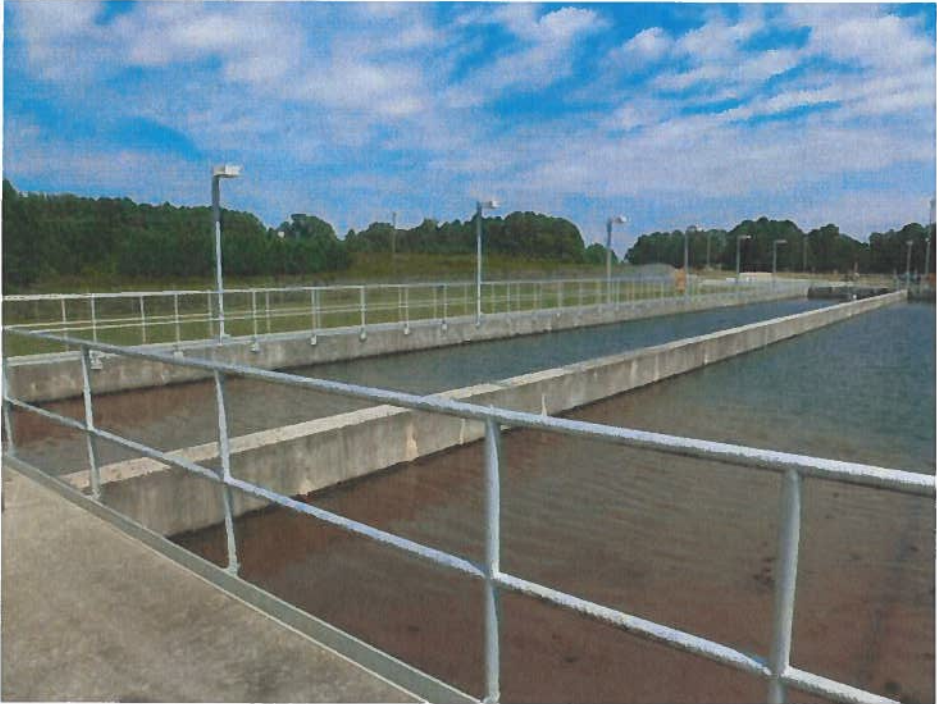
Photograph M – Sedimentation Basins
