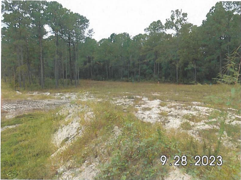
Photograph FF- Right-of-Way at US Hwy 421 from 2019 - 48" RWM Relocation Project
