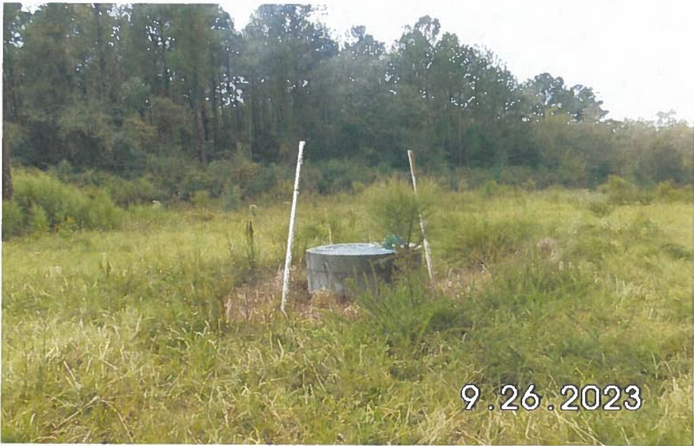
Photograph BB – Orange Painted Structure Marker Deterioration
