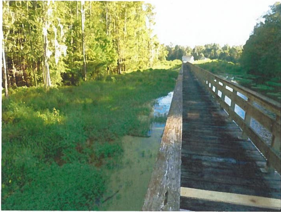
Photograph O – 60-inch Intake Pipeline Corridor
