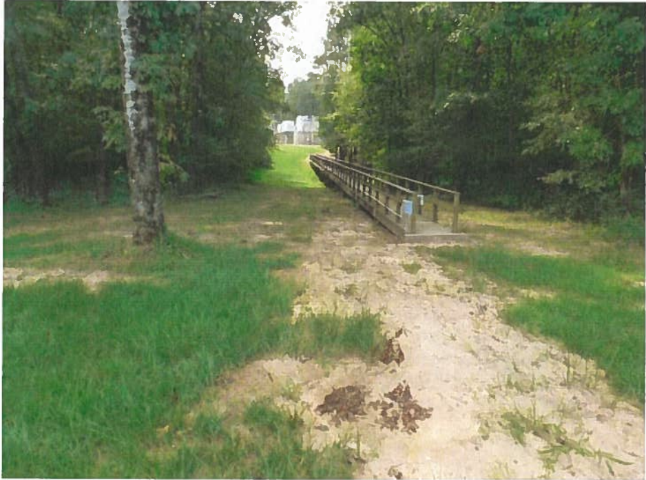
Photograph D – River Access Walkway
