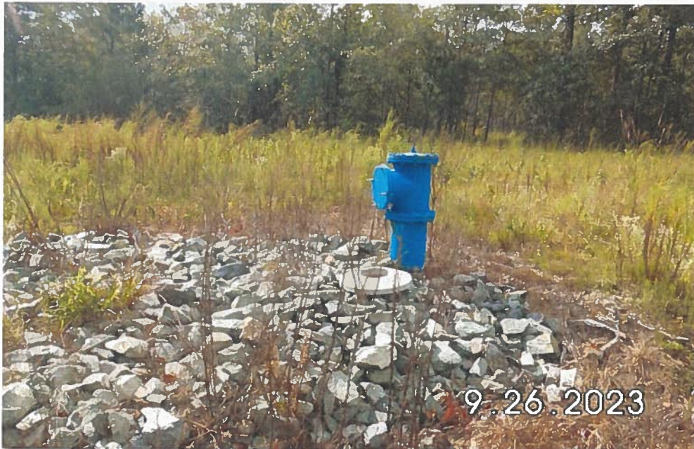
Photograph GG- Old Blow-off on 48" RWM and new Blow-off on 54" RWM
