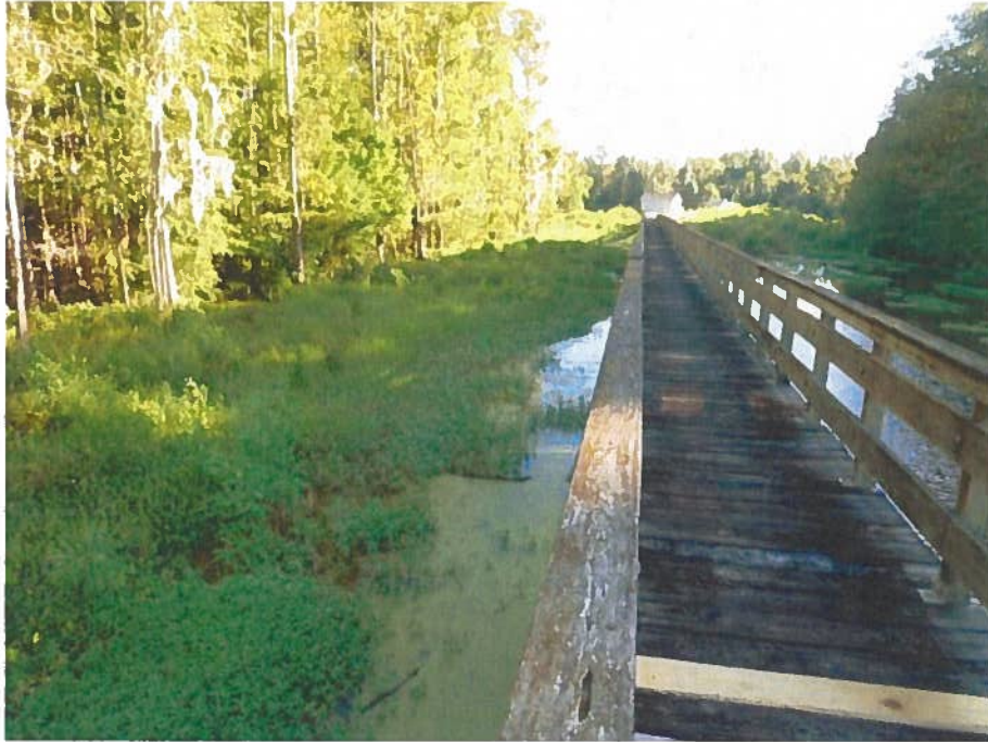
Photograph O – 60-inch Intake Pipeline Corridor
