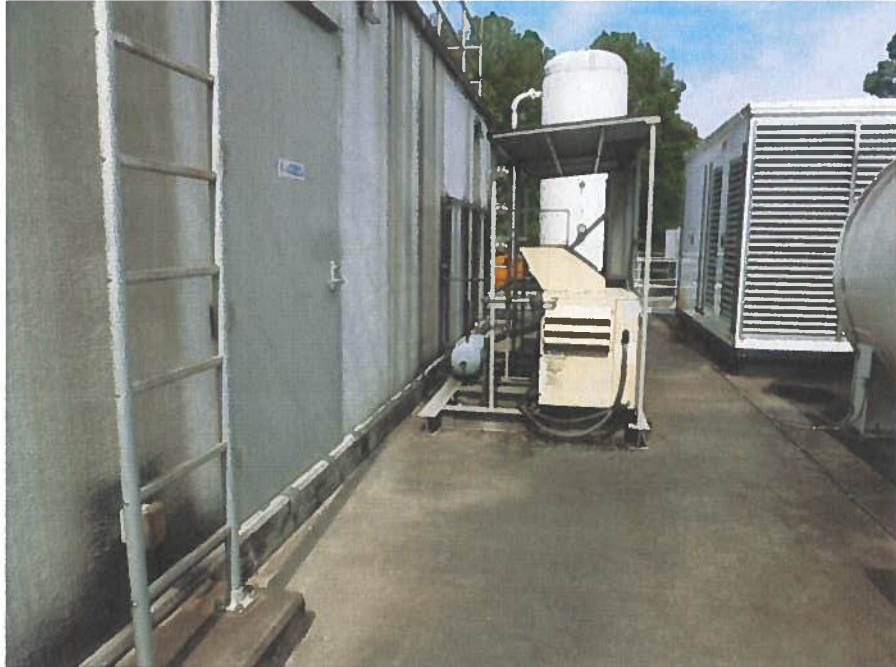
Photograph J - Restored air compressor skid support framing
