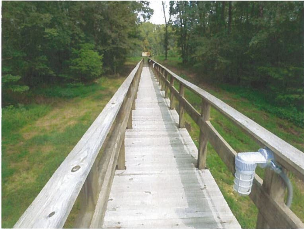
Photograph C – River Access Walkway
