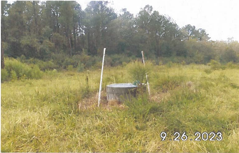
Photograph BB – Orange Painted Structure Marker Deterioration
