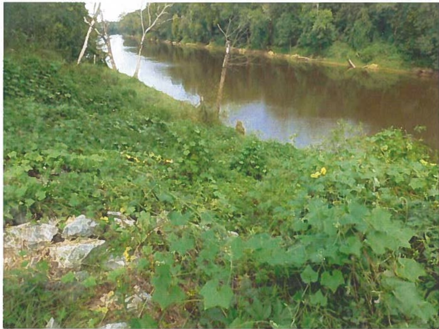
Photograph B – Cape Fear Riverbank Restoration Project Area
